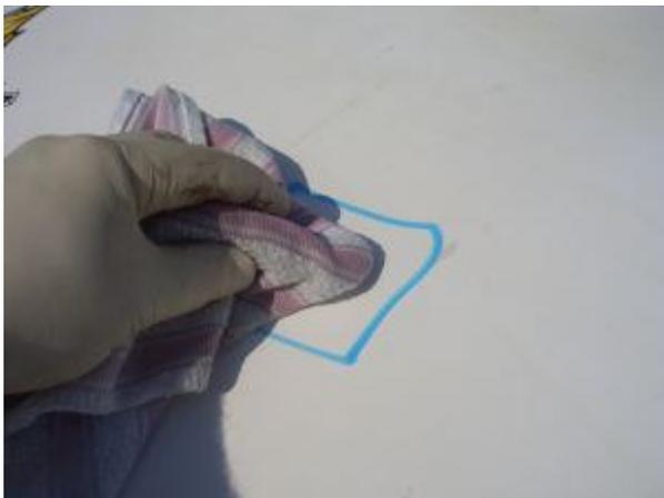
Clean off the board's surface all around the hole, using a rag soaked in alcohol.
