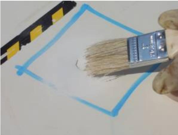
With a clean brush, wet the board surface around the hole with resin/hardener mix. This ensures that the epoxy will get a good grip on the surface of the board.
