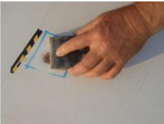
When the epoxy is fully hardened, use a sanding block and sand paper to sand the epoxy flat and level with the surface of the board.
