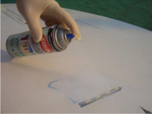
The final step is to spray paint the sanded epoxy. The paint protects the cured epoxy from UV, which will break down the epoxy if it's not shielded from the sun.
